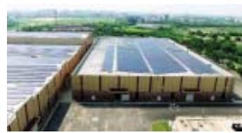
This plant, spanning across 35000 sqm of roof, consists of 7860 Trina PV modules of 320 Wp each and 33 nos. of SMA inverters.
